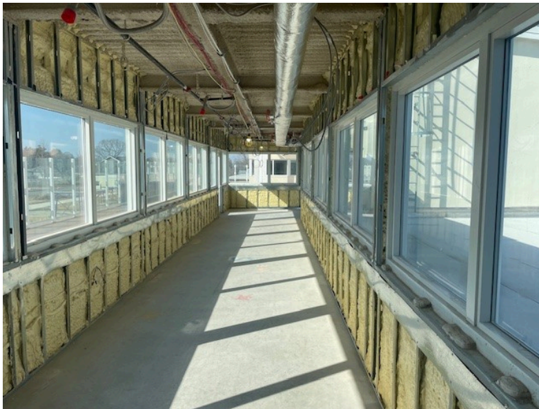
Sprayed Insulation on the 2nd floor Medicare corridor
