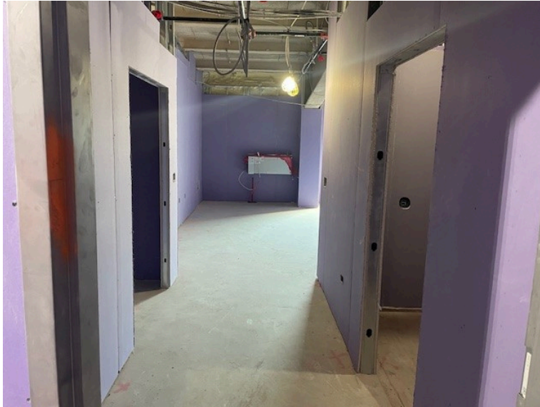
View of sheetrocked room within the West Wing's 2nd floor
