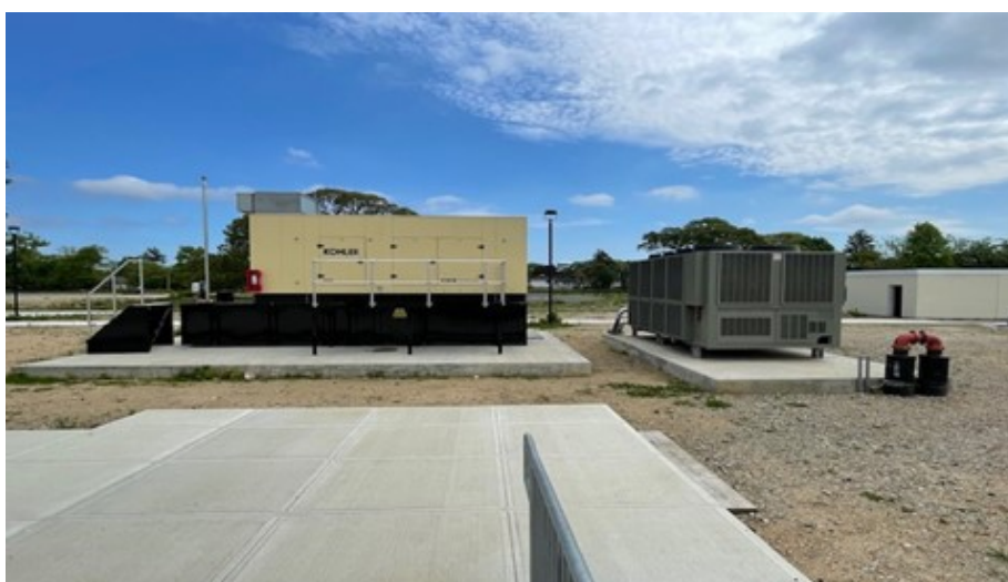
Installed chiller and emergency generator
