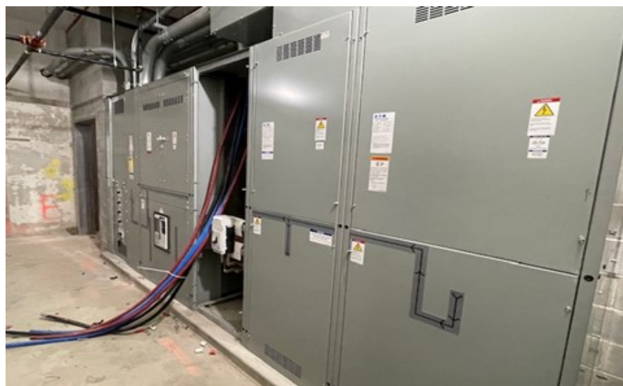
Electric switchgear room getting ready for permanent power
