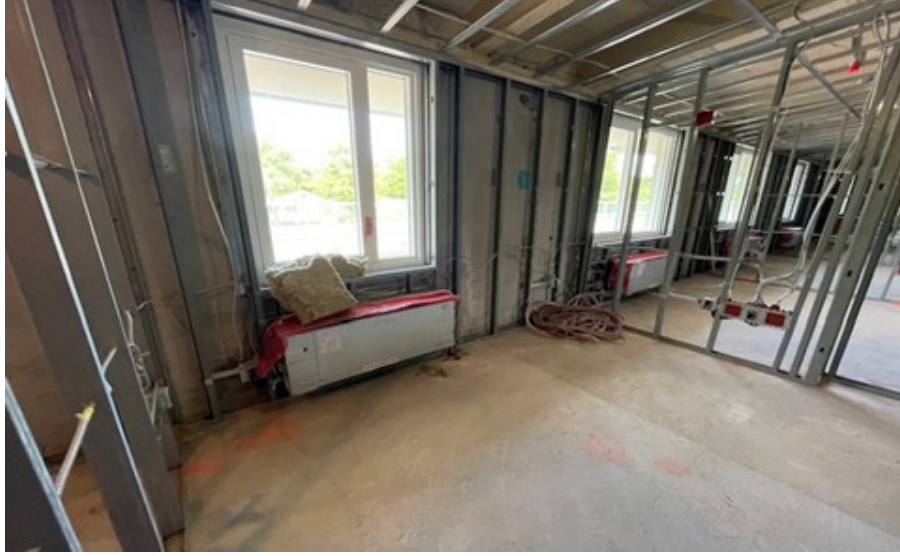
Installed individual room heating- AC units
