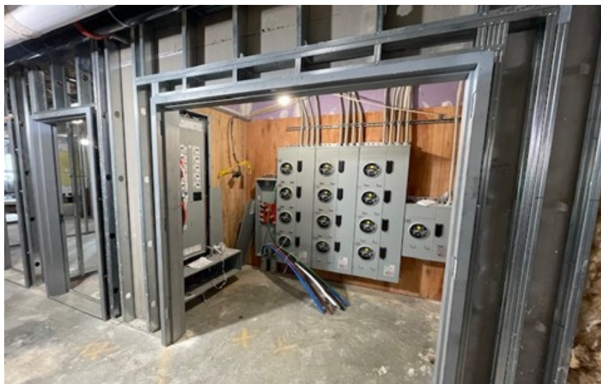
Installed electric meters for Independent Living Apartments
