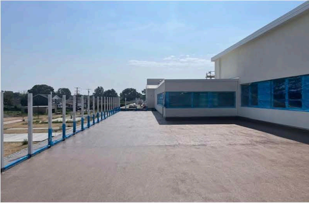
View of substantially completed framing throughout the building
