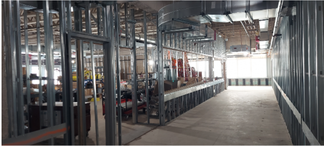
Partitioning mostly completed
