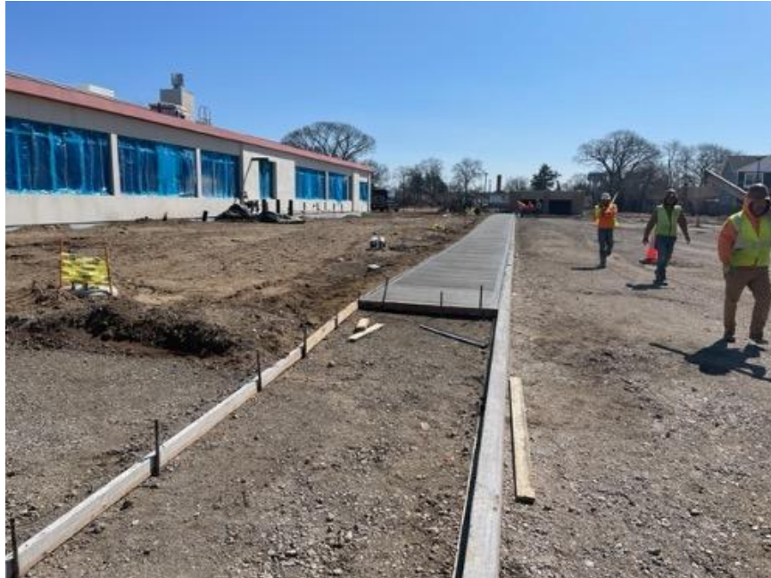
Poured concrete sidewalks along west side of the facility
