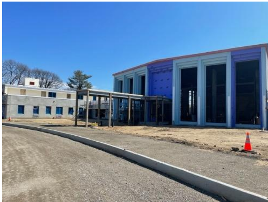
Front Elevation and Main Entrance of the Facility
