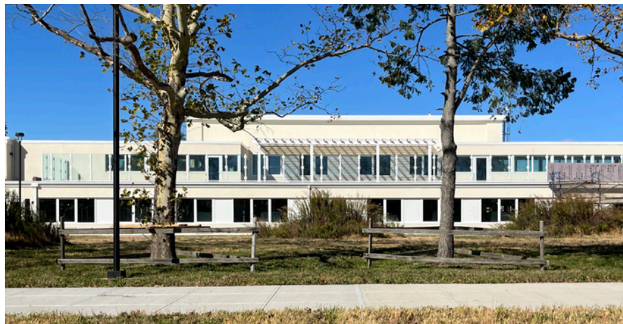
2ND FLOOR MEMORY CARE ROOF GARDEN
